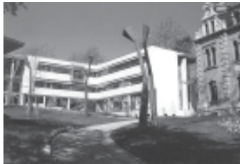
new and old building of the institute
