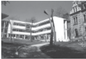
new and old building of the institute
